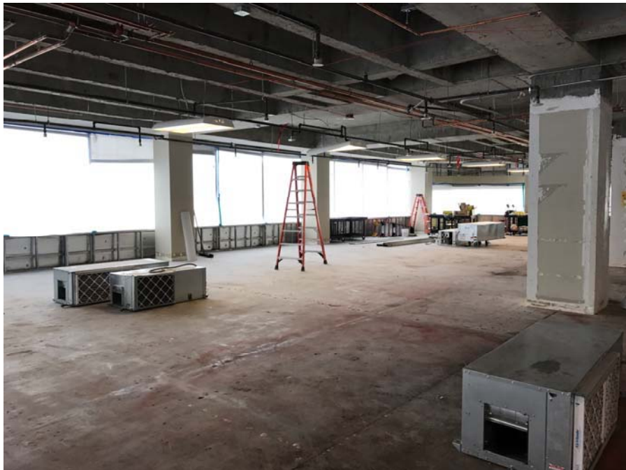
Floor immediately below the K277AE antenna
