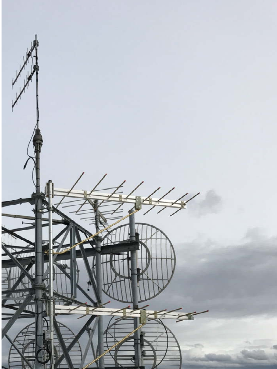
Antenna support structure. The K277AE antenna is the pair of stacked log periodic antennas located on the support structure leg closest to the camera.
