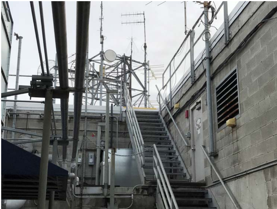
Stairwell leading to roof. K277AE antenna support structure visible on roof
