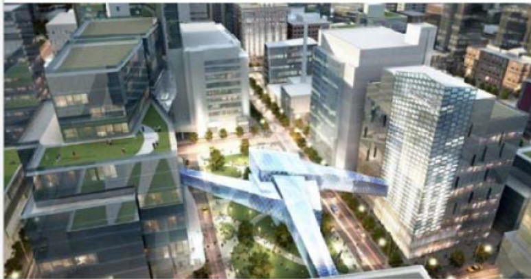
Construction Dive's 'mini megacities' to watch: Rochester, Minnesota constructiondive.com
